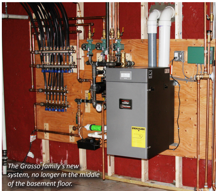
Without a convenient place to hang the boiler, Absolute precision studded out the basement wall.
