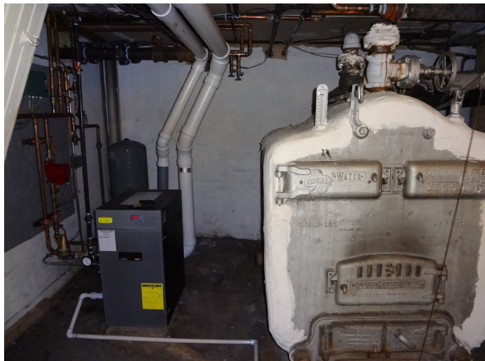
Old and new worlds collide, when a Burnham Alpine condensing boiler is installed to do the same job as the cast-iron dinosaur beside it.
