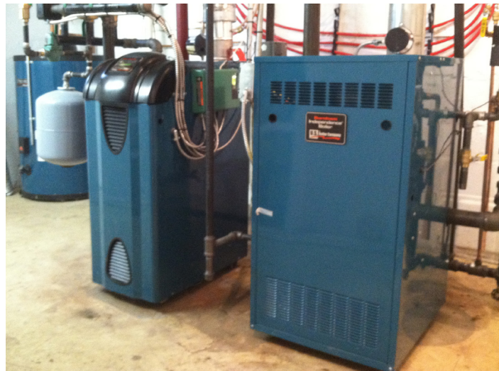
A Burnham Independence supplies steam to cast-iron radiators, while an ES2 heats in-floor zones and DHW via a Burnham Alliance sidearm tank.
