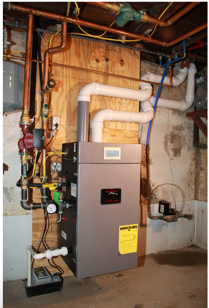
(top left) Customer Service Rep, Ellen Santiago. (top right) Office Manager, Alicia Lloyd. (bottom) For gas retrofits, Goldberg and Aire Serv techs have standardized on the Alpine condensing boiler. Here, a newly installed 105 MBH unit heats a 2-zone rancher.
