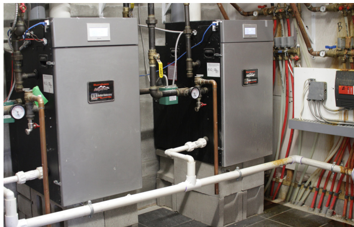
The two Alpine boilers at the King residence are elevated on cinder blocks because of the home's proximity to the river.
